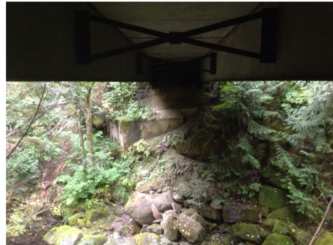
Right Bank Abutment when facing downstream
