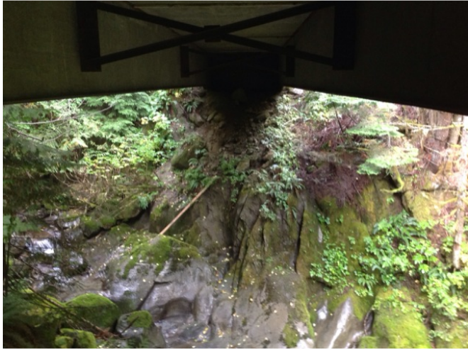
Left Bank Abutment when facing downstream
